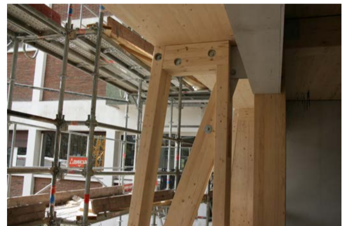
For the vertical structure of the wooden balconies.
